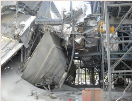
Picture 1: Collapsed ESP
